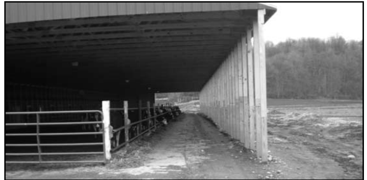
Heritage Hill Farm – Fort Ann – The Mattisons completed this roofed barnyard (right) to eliminate polluted runoff from Halfway Creek. The pollution originated from the former open barnyard (left). The project was funded through a special Southern Lake Champlain Water Quality Improvement Project through the Lake Champlain Basin Program. The work was completed by S&L Builders of Pennsylvania.
